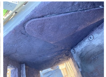
New flopgate coated with Belzona Ceramic Carbide FP (1812)
