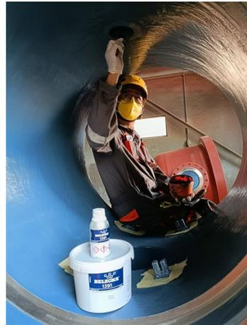
Belzona 1391 brush applied in a nozzle.
