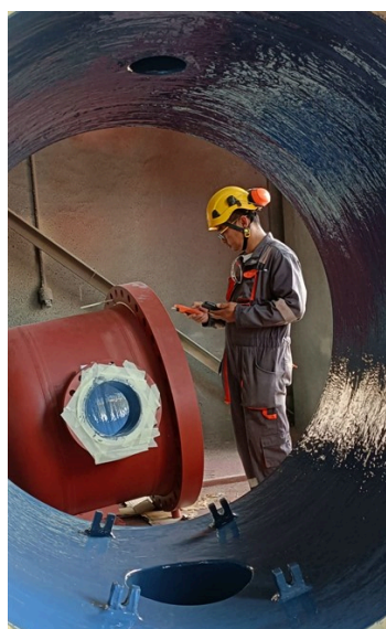
Overall internal surfaces coated with Belzona 1391.
