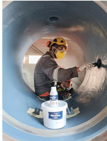
Belzona 1391 brush applied in a nozzle.
