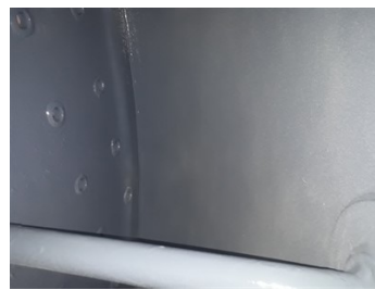
Initial coat of Belzona 1321 being applied
