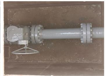
Pipeline fully coated for corrosion protection
