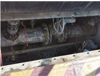
Original condition of the corroded pipeline
