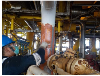
Applying 3 coats of Belzona 5871 by brush
