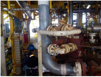
Surface preparation with hand tools on bare metal after aluminium cladding removal
