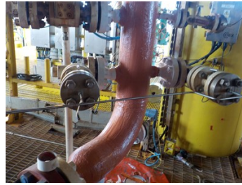
Leave the applied coating to expand by foaming and cure
