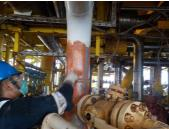
Surface preparation with hand Applying 3 coats of Belzona 5871 by brush
