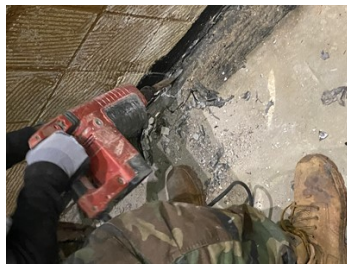
Preparing the surface
