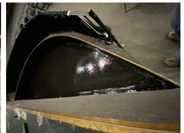
5811 top coat was applied
