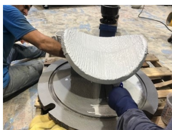
Priming coat of Belzona 1331
