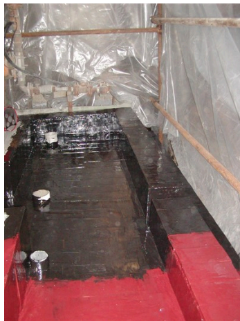
Protection of chemical containment area in progress
