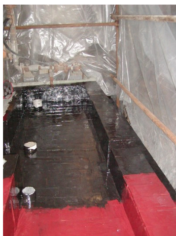
Protection of chemical containment area in progress
