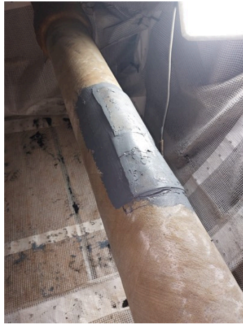
Steel plate bonded over the hole with Belzona 1212
