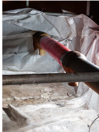
Damaged area reinforced using Belzona Super Wrap 2
