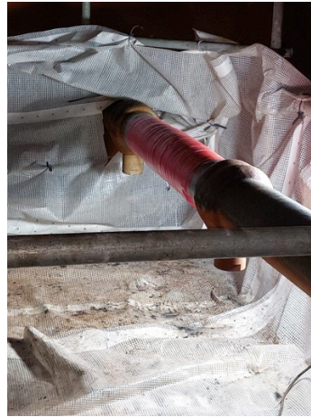
Damaged area reinforced using Belzona Super Wrap 2
