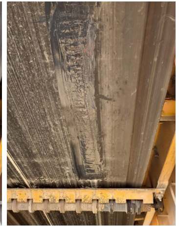
Belt fasteners protected with Belzona 2311
