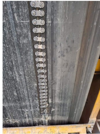
Belt fasteners installed
