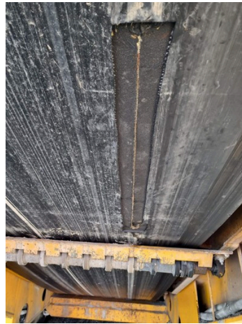
First layer of the belt peeled off in order to install belt fasteners properly
