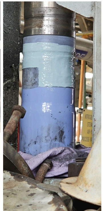
Belzona 1593 (high temperature coating) applied to seal the area.
