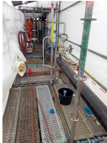
First 5 meters of Belzona SuperWrap completed. 35 meter to go.
