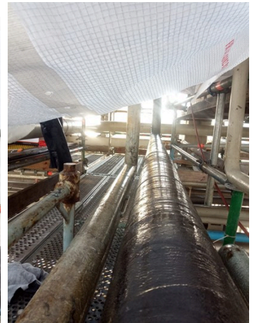
Finished application halfway the pipe.
