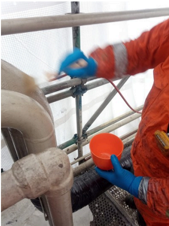
Surface preparation. A thin layer of Belzona 1983 onto the pipe.
