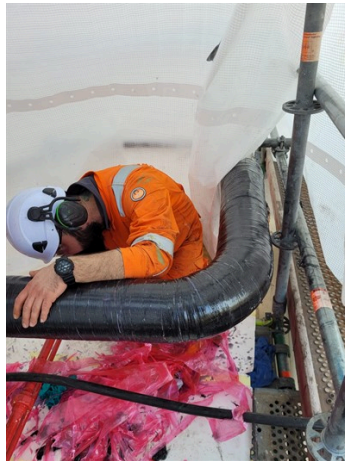
After curing removing the Belzona 9382 tape to inspect the application
