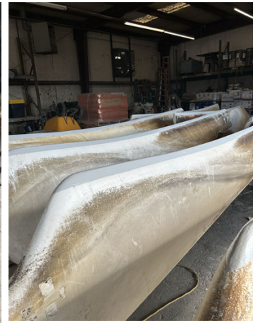
Completed View 2 - 4" Strip of Belzona 5721 Applied to Leading Edge
