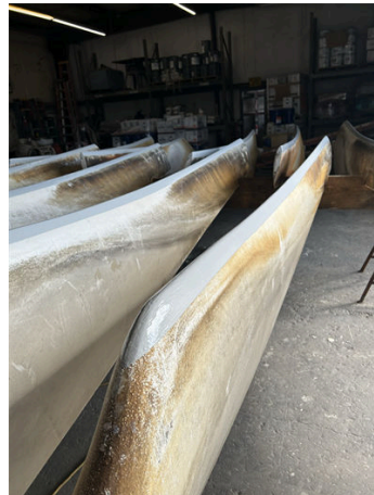
Completed View 1 4" Strip of Belzona 5721 Applied to Leading Edge
