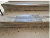
Loss of thickness on a stair due A stair rebuilt to its original to 120 years of wear, level using Belzona 4111 represents a risk of falling and injury.
