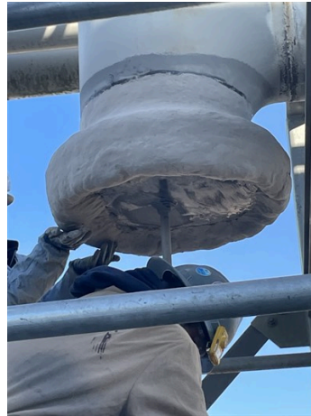
Encapsulation of entire head.
