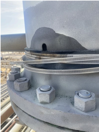
Line clamp leaking.
