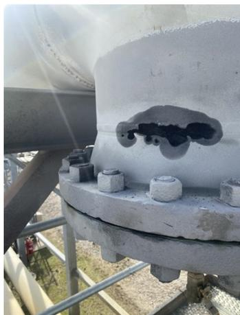
Clamp removed and vapor blaster used.
