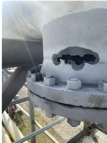
Clamp removed and vapor blaster used.
