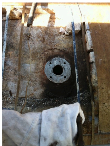
Gasket damage
