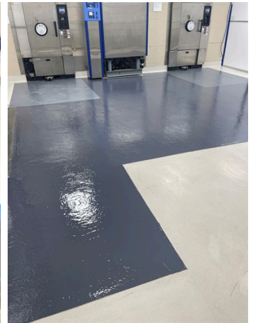
Belzona 4311 applied to rest of the area
