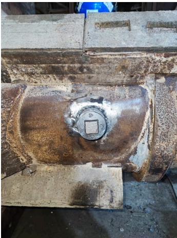
Area prepared using a power tool (MBX Bristle Blaster)
