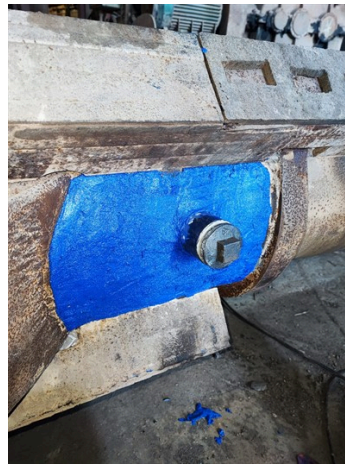
Belzona 1818 applied
