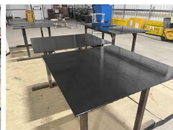
All steel work protection completed.
