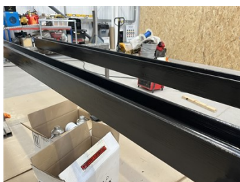
Belzona 4351 (Magma CR5) applied to supporting beams
