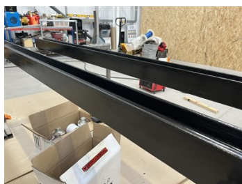
Belzona 4351 (Magma CR5) applied to supporting beams
