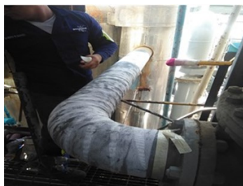
First layer of Belzona 1161 and reinforcement mesh.
