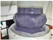
Post-application of 5x wraps of Final application after a further encapsulating layer of Belzona
