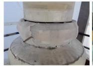
SF6 flange following surface preparation to SSPC-SP11, installation of the Backing Rod, tape, Redirection Nozzle & Breather Membrane.
