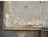
All loose material removed and Belzona 4911 Conditioner the surface prepared with a hand grinder on both the concrete surfaces and metal surfaces.
