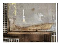
Previous failed repair material removed.
