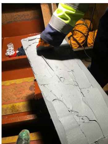
Belzona 1111 applied to plate
