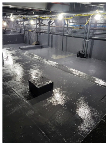
Final coat of Belzona 4311
