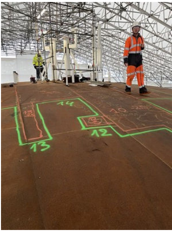
Roof prior to the application.
