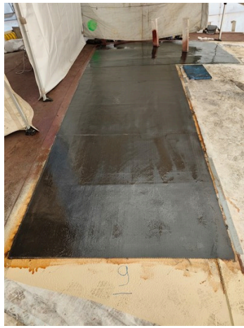
Application of the first layer.
