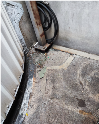
Clears signs of chemical damage on bund floor
