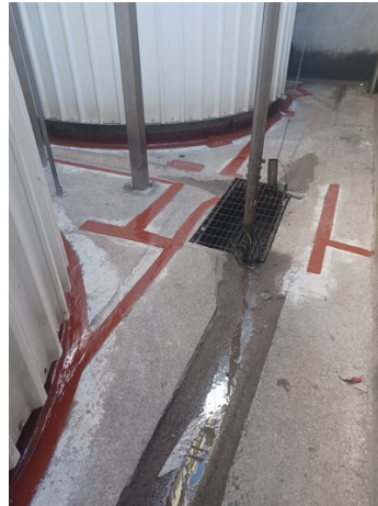
Repairs with 4131 and sealing of cracks with 4361
