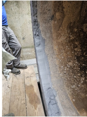
Rebuilding the damage using Belzona 1111.
