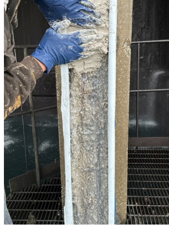
Application of Belzona 4141 for repair
