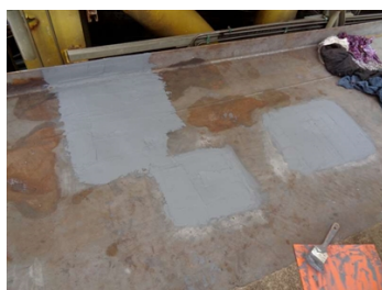
Fixing the holes with Belzona 1161 and re-inforcement sheets
