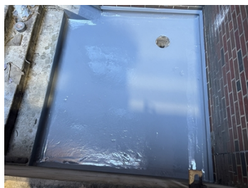
Belzona 5811 as our base coat to the "basin"
