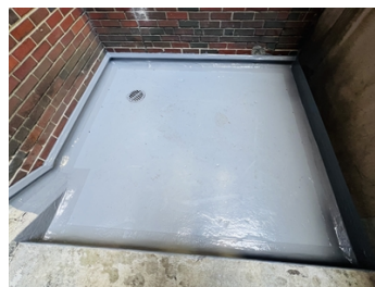
Belzona 3121 with Reinforcement cloth to the seams
