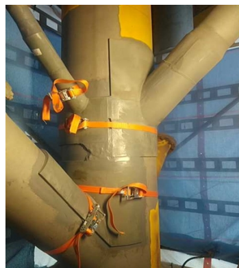
Bonding custom made reinforcement plates.
