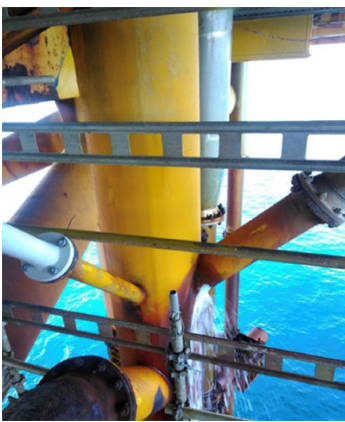
Severe corrosion on 24" caisson.
