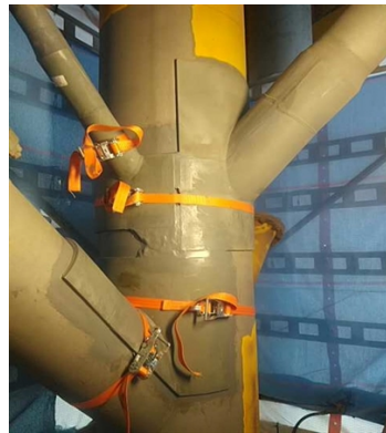
Bonding custom made reinforcement plates.
