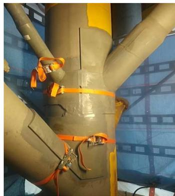
Bonding custom made reinforcement plates.
