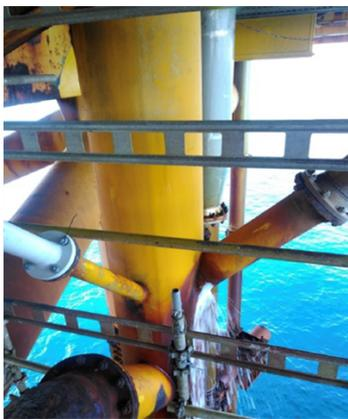
Severe corrosion on 24" caisson.
