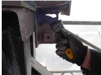
Surface preparation & wetting out with Belzona 7311
