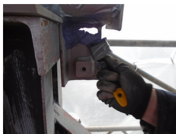
Surface preparation & wetting out with Belzona 7311
