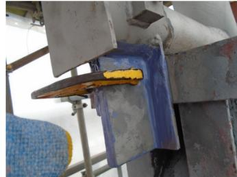
Doubler plates installed & clamped in place
