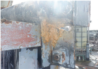
Corroded section covered in wax oil
