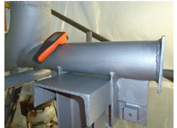
Completed repair overcoated
