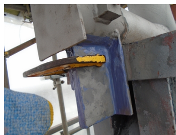
Doubler plates installed & clamped in place
