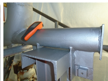
Completed repair overcoated
