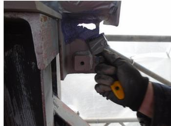
Surface preparation & wetting out with Belzona 7311
