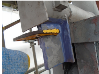
Doubler plates installed & clamped in place
