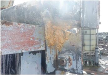
Corroded section covered in wax oil
