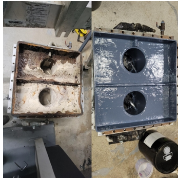
Before and after Belzona application
