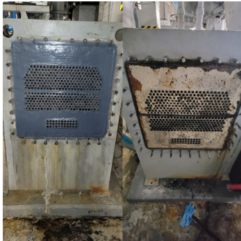
Before and after Belzona application
