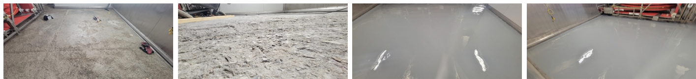
Area prior to application Commencement of application Belzona 5811 applied to area Application completed
