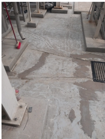
Cracks in concrete of bund area
