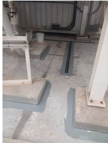
Cracks in concrete of bund area Prepared edges of plinths
