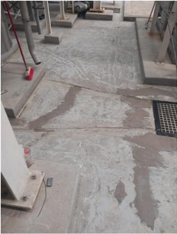
Cracks in concrete of bund area
