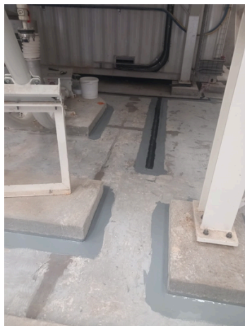
Prepared edges of plinths
