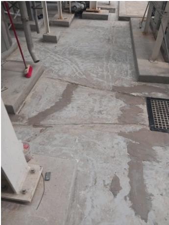
Cracks in concrete of bund area Prepared edges of plinths
