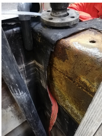
Ebonite tank suffering from degradation
