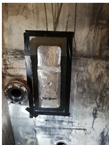
Surface prepared and area taped off, ready for application
