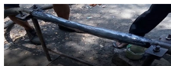
Finished application with Belzona 2211 (MP Hi-Build Elastomer) applied on the damaged areas.
