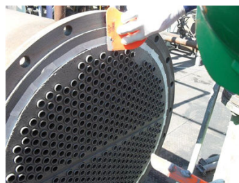
3.) Applying Belzona 1111 for the rebuild
