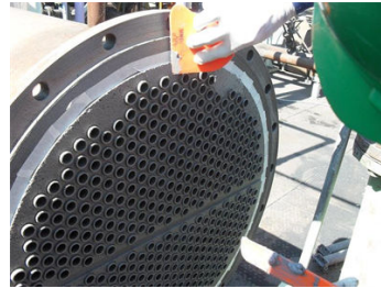
3.) Applying Belzona 1111 for the rebuild
