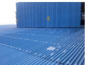
Tin roof required a repair on anchor bolts and joints to prevent water ingress
