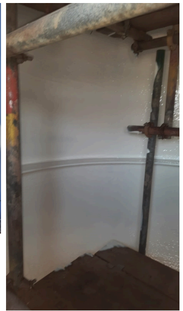
Protected tank interior after application
