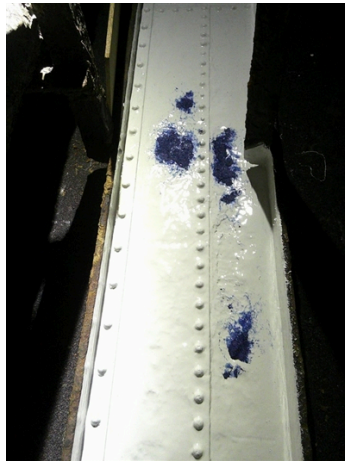
First coated throughout with Belzona 5831LT and pit filled with Belzona 1818
