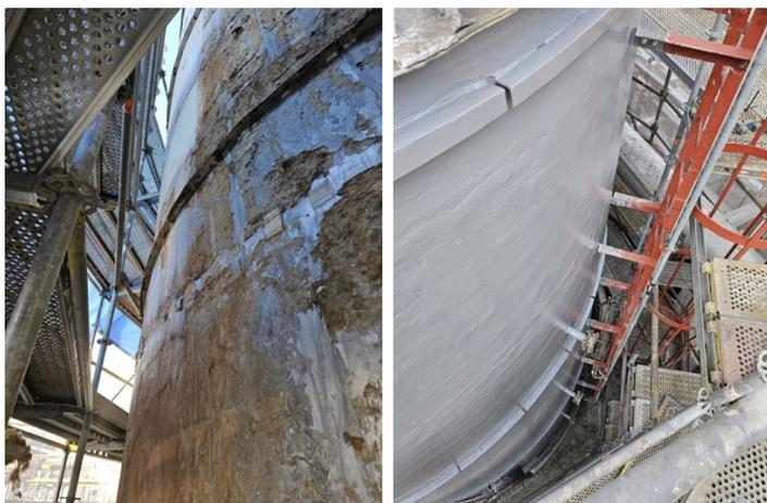
Tank walls damaged caused by corrosion      Finished application
