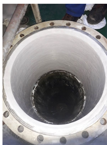
Finished application after two coats of Belzona 1391T
