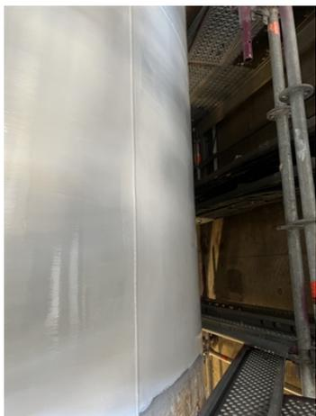
First coat of Belzona 5892 in white.
