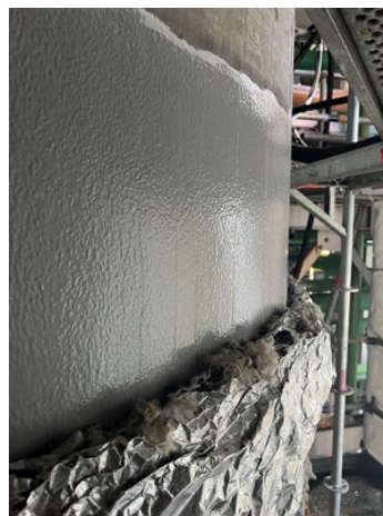
Completed coating with insulation reinstalled.
