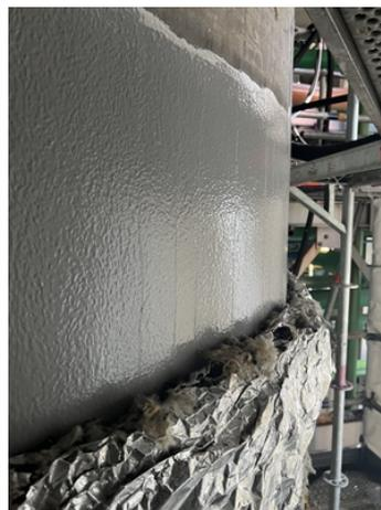
Completed coating with insulation reinstalled.
