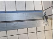
The application area was marked with tape to delimit the application area. A backer rod was inserted into the joint prior to the application of Belzona 2211.
