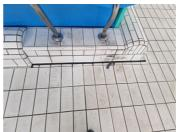
Belzona 2211 filled the expansion joint, safeguarding the concrete structure underneath from further damage.
