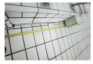
Measurement of the defective expansion joint in order to calculate the required quantity of product.
