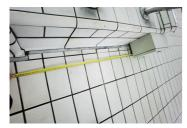
Measurement of the defective expansion joint in order to calculate the required quantity of product.
