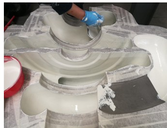
During application of Belzona 5811 DW2
