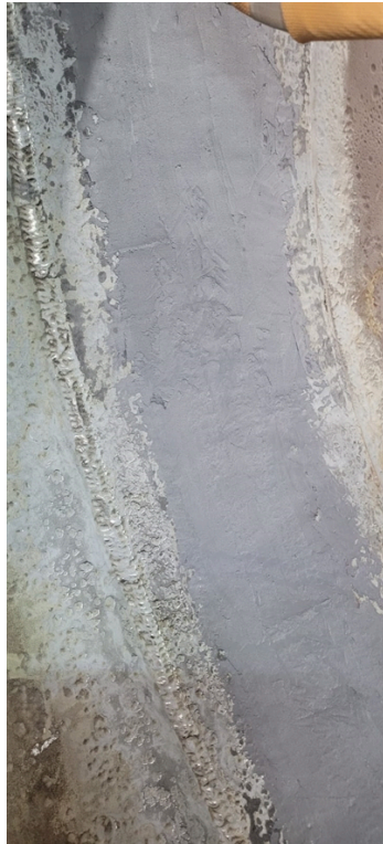
After surface preparation and rebuilding with Belzona 1311
