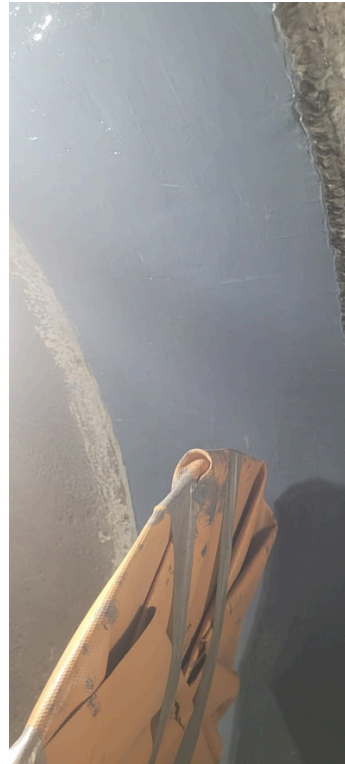
With first coat of Belzona 1321
