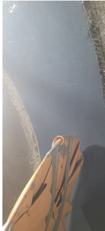
With first coat of Belzona 1321
