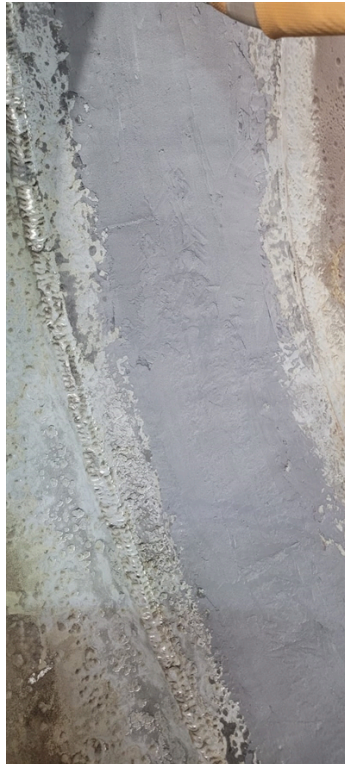
After surface preparation and rebuilding with Belzona 1311
