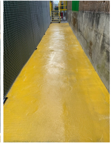
Belzona 5231 applied to half of the high traffic area
