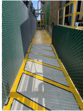
Belzona 5231 applied to half of the high traffic area
