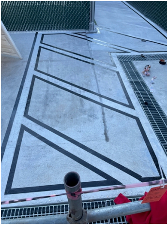
Pre Job inspection
