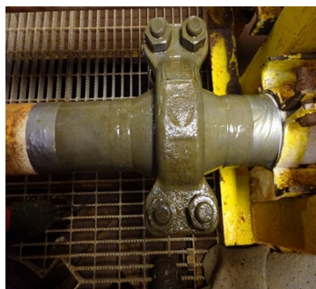
Surface preparation & Belzona 8411 applied
