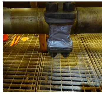
Bridging tape applied around voids
