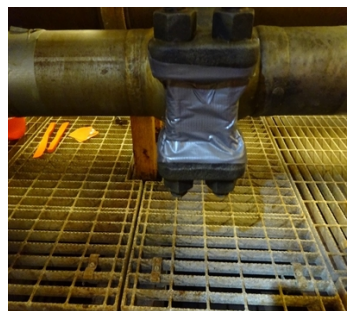
Bridging tape applied around voids
