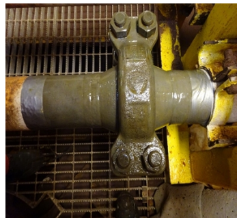
Surface preparation & Belzona 8411 applied
