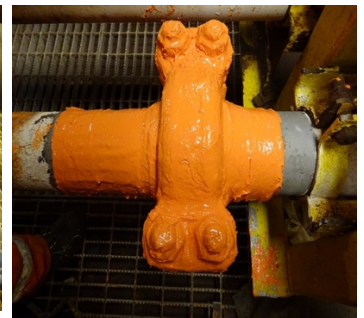
Two coats of Belzona 3412 applied
