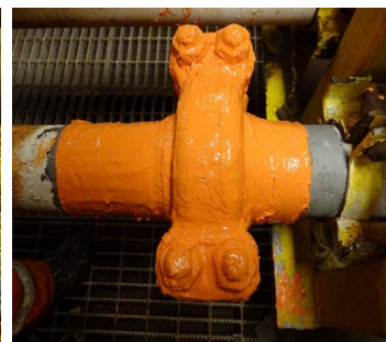
Two coats of Belzona 3412 applied
