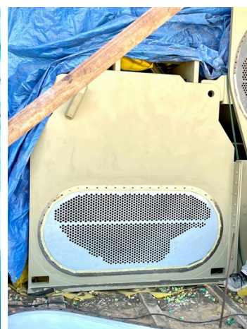
Chiller after Belzona 1321 and Belzona 1341 applications.
