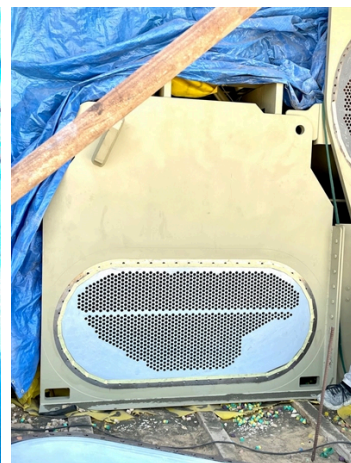
Chiller after Belzona 1321 and Belzona 1341 applications.
